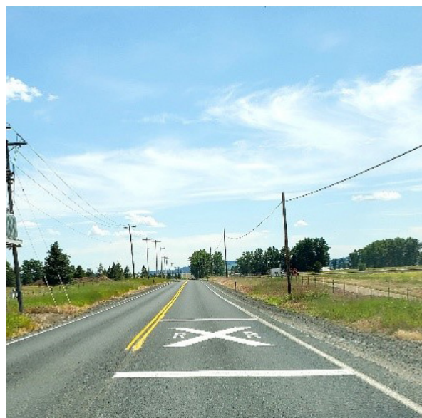
Phase 1 Rail Crossing at Craig Road
