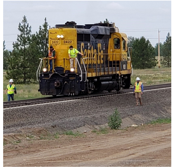
Recent Phase 1 Rail Testing
