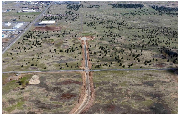
Phase 1 Construction Rail Spur
