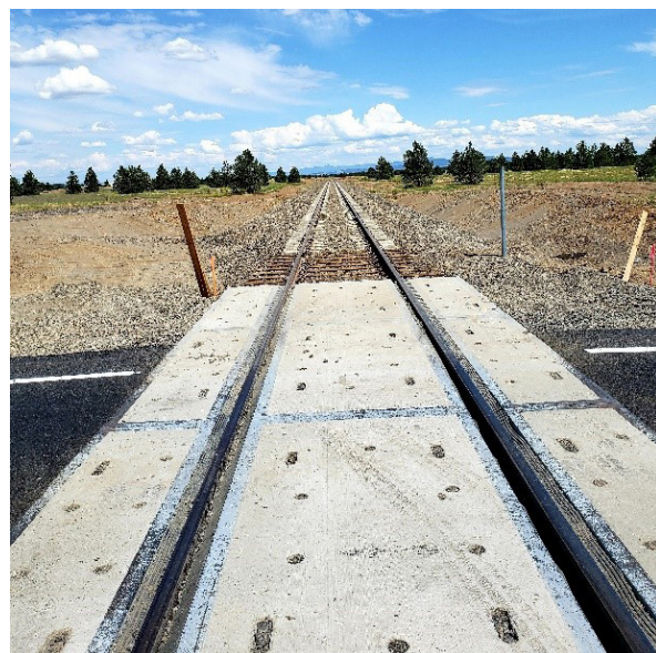
Phase 1 Rail Spur at Craig Road
