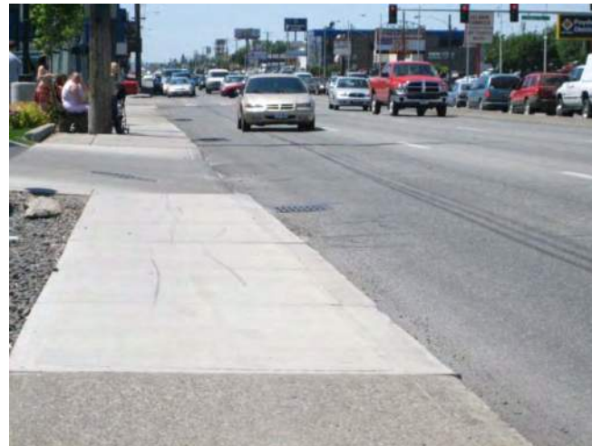
Figure 3-D: Sprague Avenue with 7-lane street section
