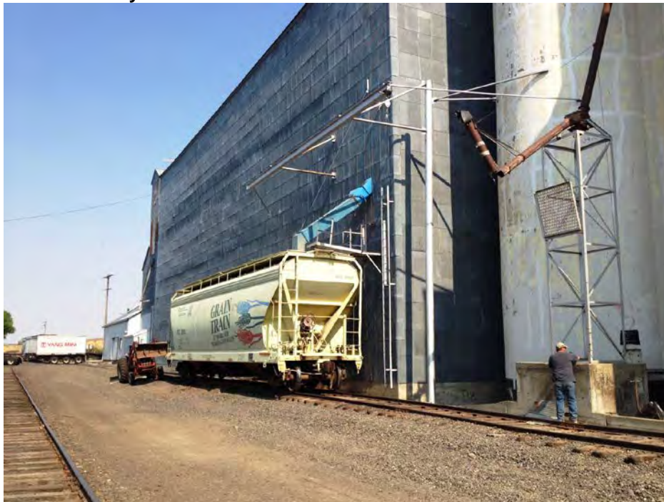
Figure 4.1: WhitGro Facility in St. John
