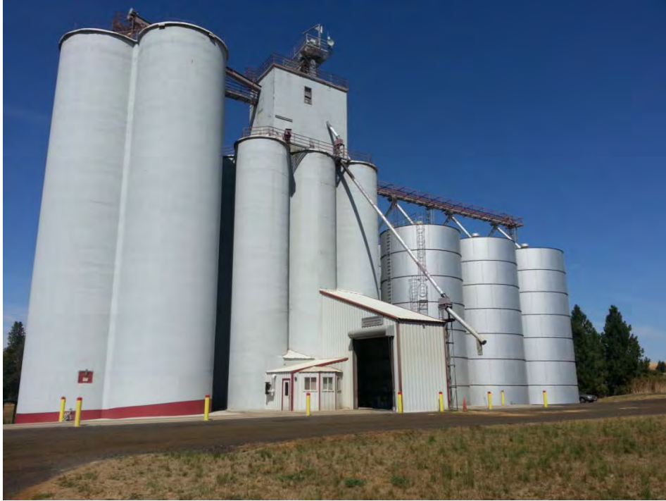
Figure 4.2: Palouse Grain Growers Facility
