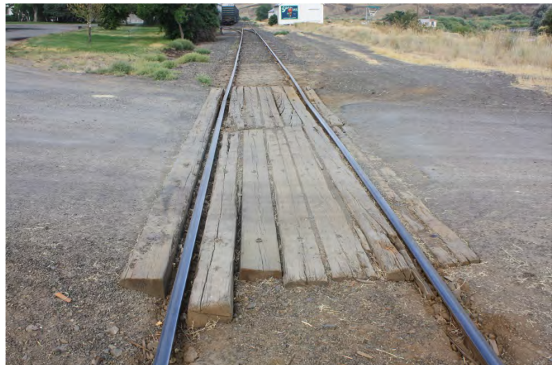
Figure 3.9: Typical Timber Plank Crossing on Hooper Branch
