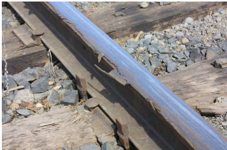
Figure 3.2: Rail Deterioration
