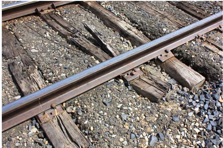
Figure 3.3: Ties on the CW Branch
