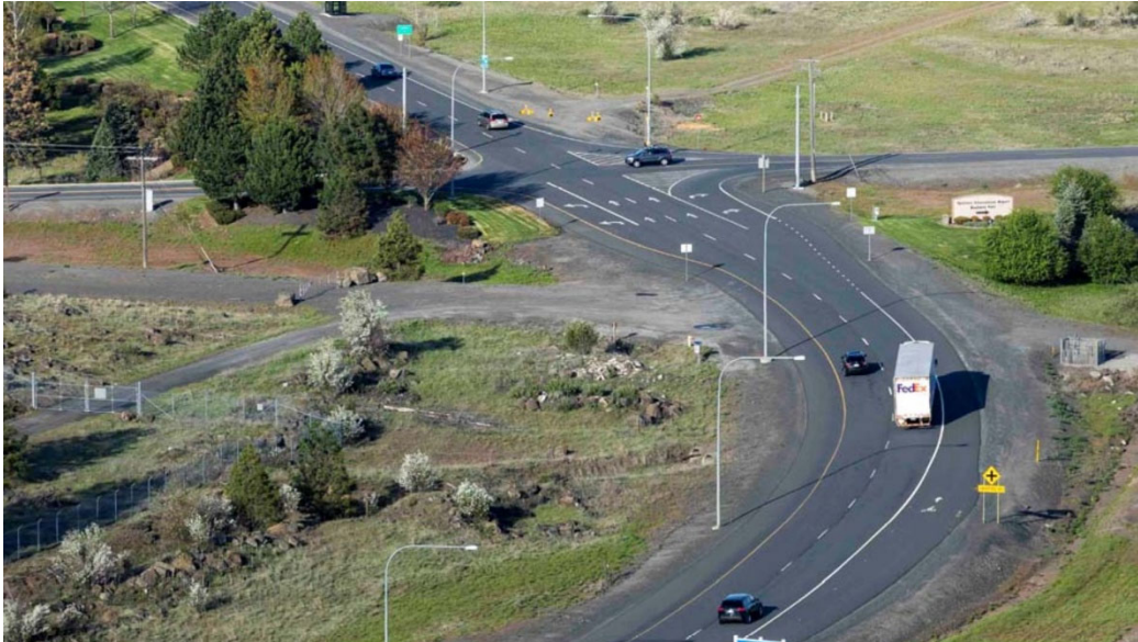
Photograph 1. Airport Drive Outbound crossing at Spotted Road.
